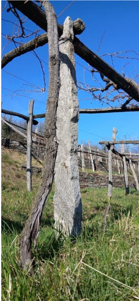
A culogna of local gneiss supporting the vine pergola.
